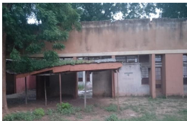
Figure 3 Bad portion of roof & finishes
