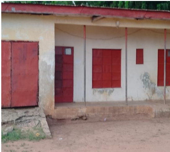
Figure 1 Bad portion of floor
