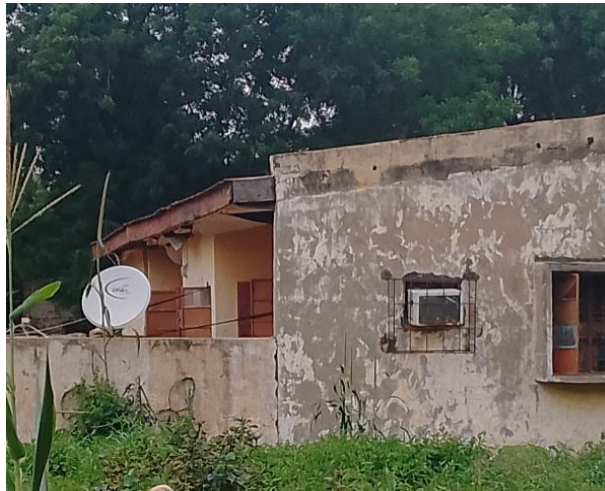
Figure 2 Paint discoloration
